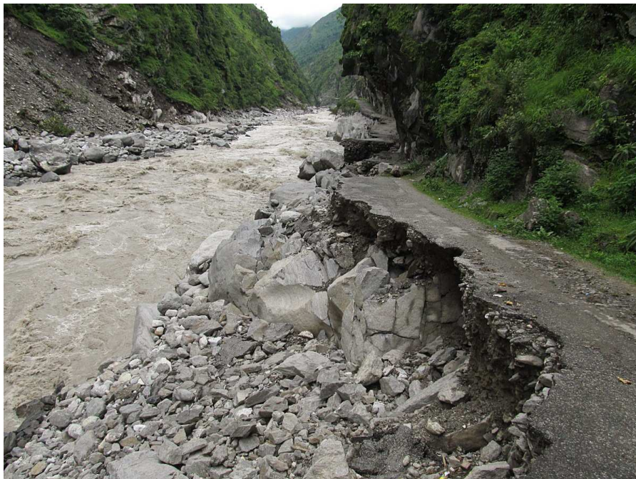
Figure 4: Section of the motor road below Tawaghat(7th July 2013 )
