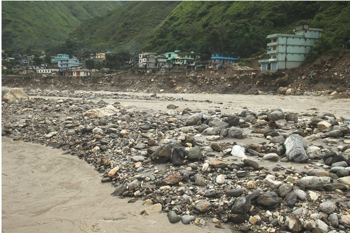
Figure 1: Khalanga Bazaar severely affected by the flooding Mahakali, Darchula Nepal, (6 July 2013)
