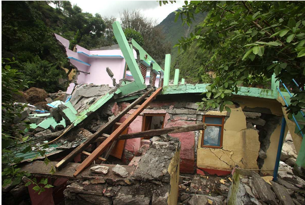
Figure 3: Completely destroyed homes at Tawaghat (7th July 2013 )
